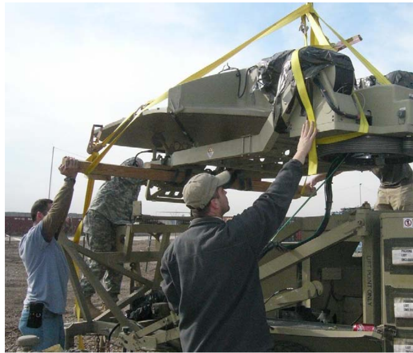
DataPath Field Engineers working with soldiers from the U.S. Army’s 2 nd Brigade, 2 nd Infantry Division to repair an STT that was damaged in a direct mortar hit in Iraq.
